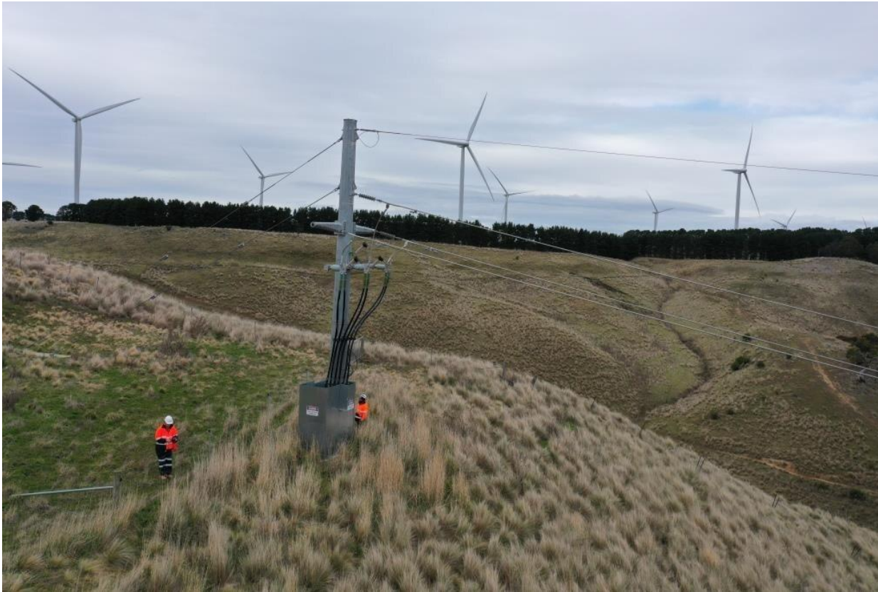
Eastern Tower Structure - 33kV Overhead Line
