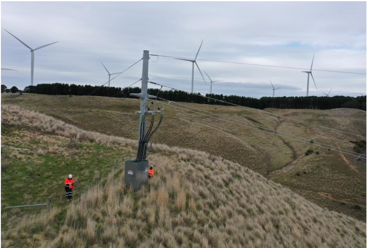
Eastern Tower Structure - 33kV Overhead Line
