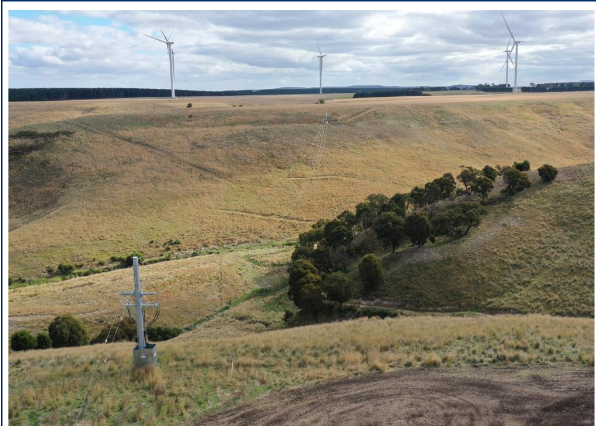
Plate 2 – View west from Eastern Tower showing clearance from trees
