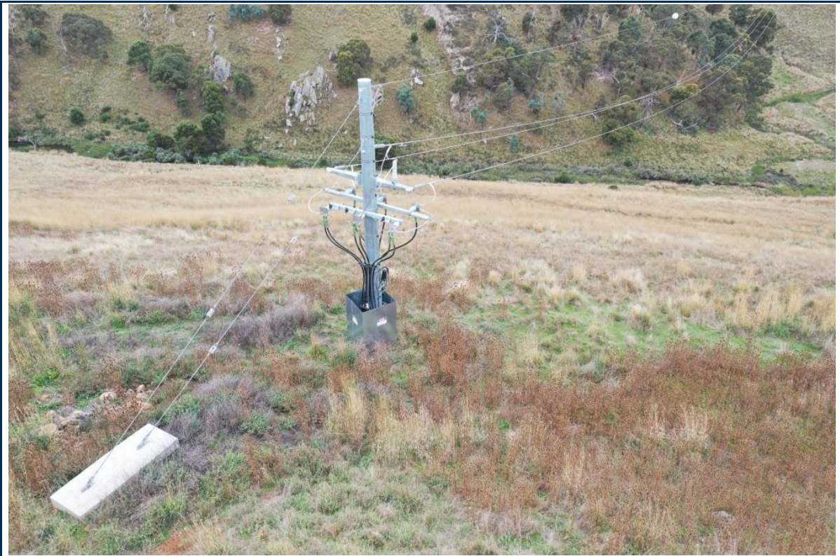
Plate 7 – Western Tower 33kV overhead line, Weeds appear to have been treated
