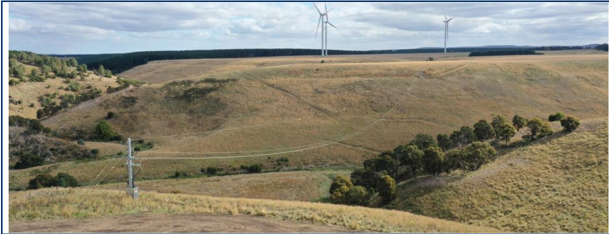
Plate 1.– 33kV Overhead line spanning MREB, Single Tower each side of the span
