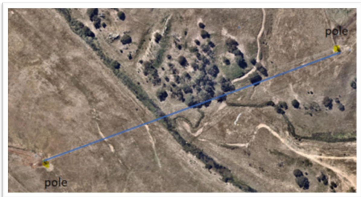
Figure 0-1 location of the Overhead line and poles across the Moorabool River East Branch
