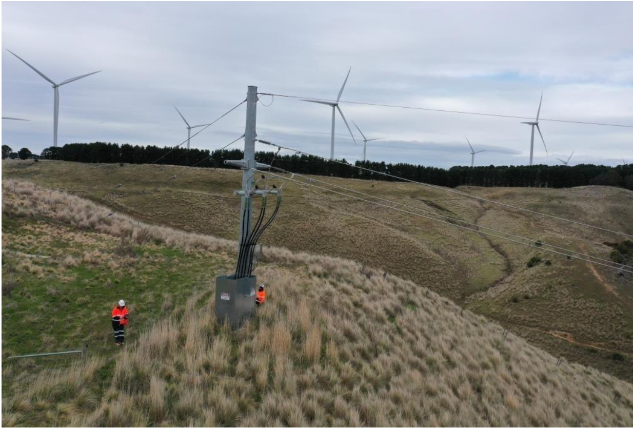
Eastern Tower Structure - 33kV Overhead Line
