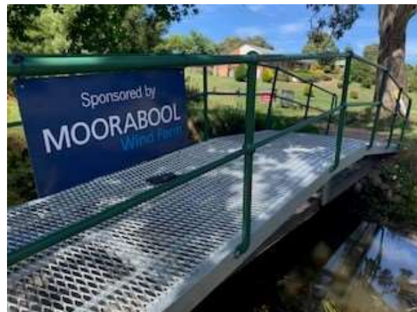
Replacement Bridges at Ballan Golf Club – Funding provided by MWF community fund Round One 2020.
