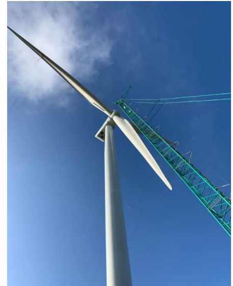
Image – Installation of Turbine 15 at MSWF
