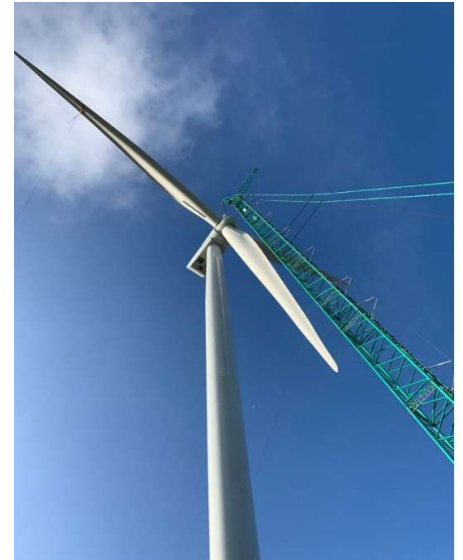
Image – Installation of Turbine 15 at MSWF
