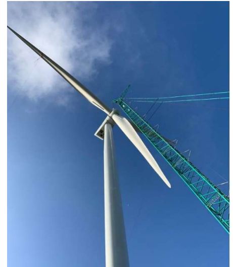
Image – Installation of Turbine 15 at MSWF
