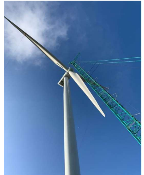
Image – Installation of Turbine 15 at MSWF
