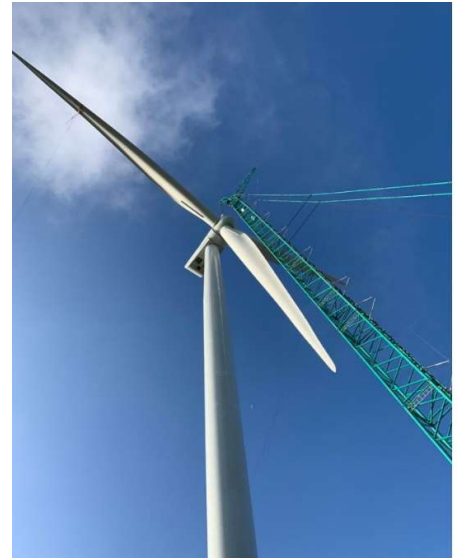
Image – Installation of Turbine 15 at MSWF
