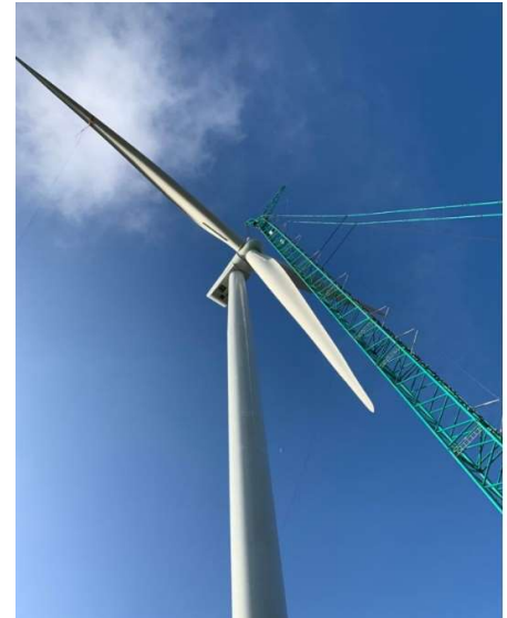
Image – Installation of Turbine 15 at MSWF
