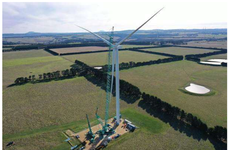
Image - Installation of the first turbine at Moorabool South wind farm
