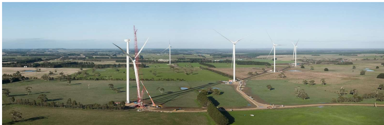
Figure 1: MNWF Rotor lift
