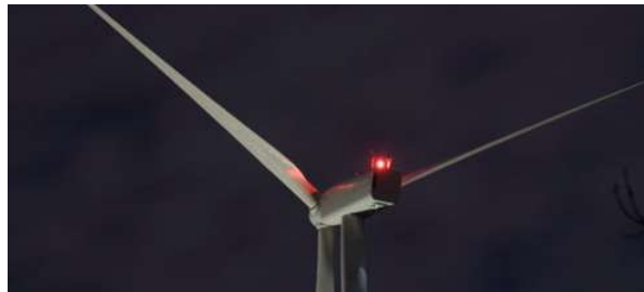
Image 1: Example of Aviation Warning Light for Moorabool Wind Farm
