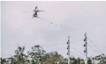
Helicopter stringing took place at 2 sections of the wind farm. Heli-stringing is much quicker and less impactful than traditional methods.
