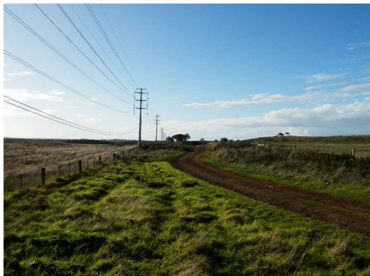
Photograph shows a typical double circuit pole during conductor stringing construction
